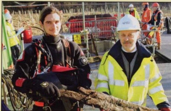
Deep debris: Structural Engineer Dave Wood (right) and Diver Mark Manning examine material from the shafts
