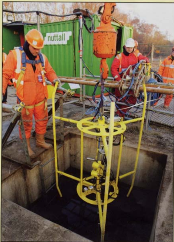
Down under: The shaft inspection system is lowered
