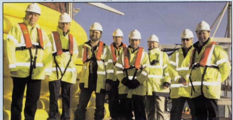
On board: Project team take a close look at the repair operation
