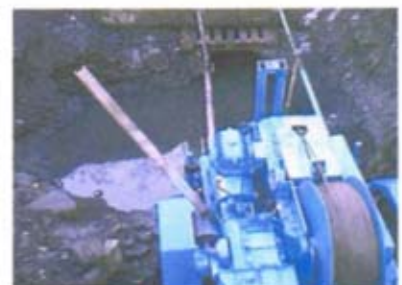
Cleaning a Culvert of blockages
