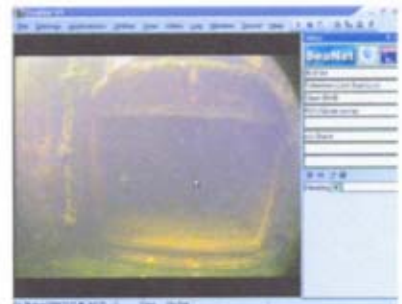
CCTV of Lock Gate Sluice Culvert
