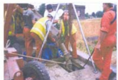
Grout Injection to stabilise Pipe
